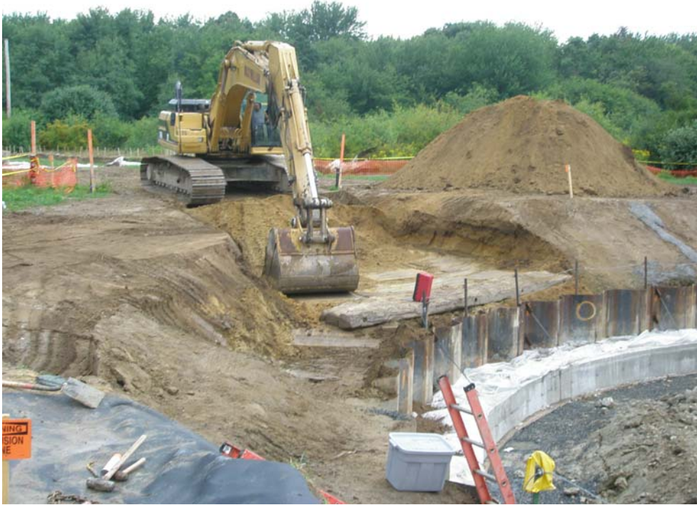
Photograph 1 – Excavation of Northeast Corner for Equipment Positioning
