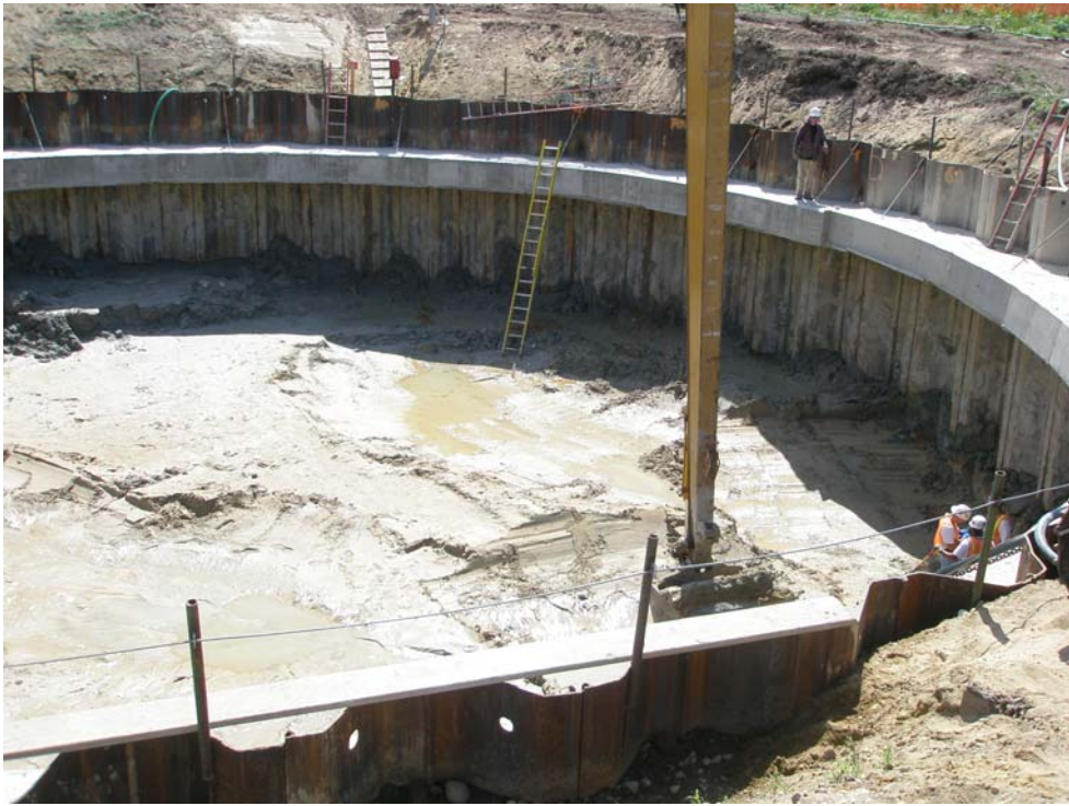
Photograph 5 – Excavation of Areas Likely Contaminated Below 107' asl
