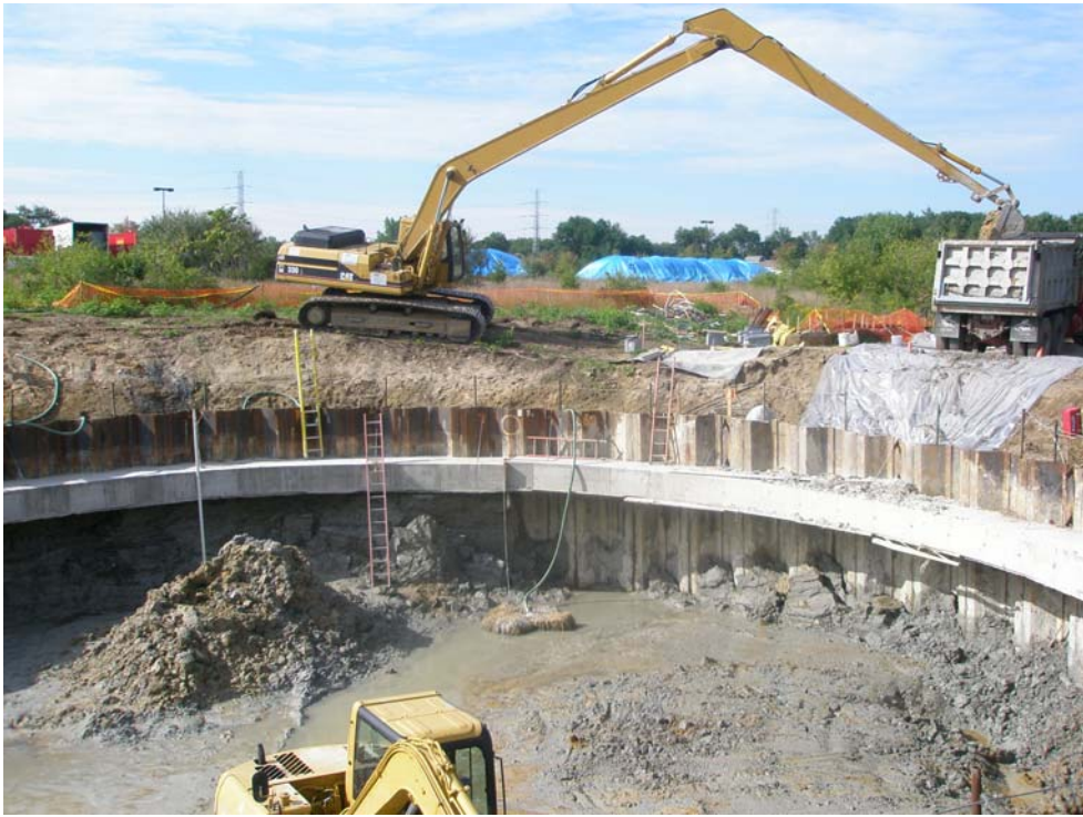
Photograph 3 – Transportation of Soil from Excavation
