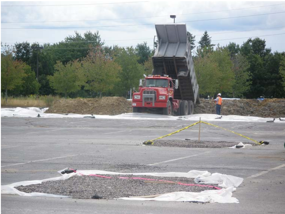
Photograph 4 – Transportation of Soil to Staging Area in Parking Lot
