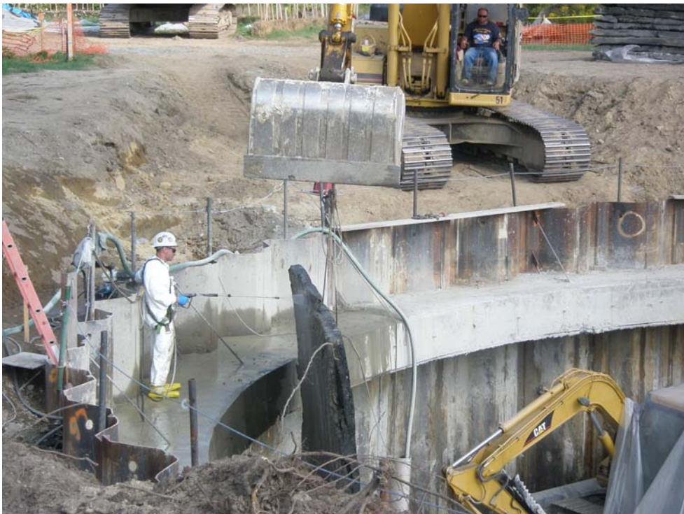
Photograph 6 – Pressure-Washing Tundra Mats in Preparation for Removal from Excavation
