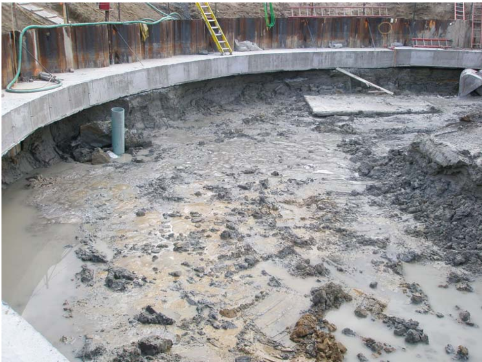
Photograph 2 – Beginning of Excavation to 107' asl, Installation of Sump
